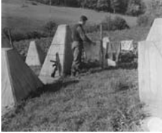
Wikimedia Commons U.S. Army Signal Corps Photographer: Wescott.. Putting out washing on the Siegfried Line15 September 1944
